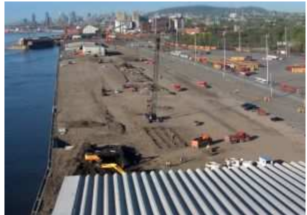
Montreal's 18.8-hectare Viau sector is being converted to handle boxes
