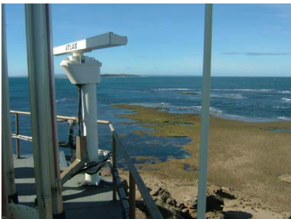
Figure 6 View of the radar antenna at Pt. Lonsdale Lighthouse
