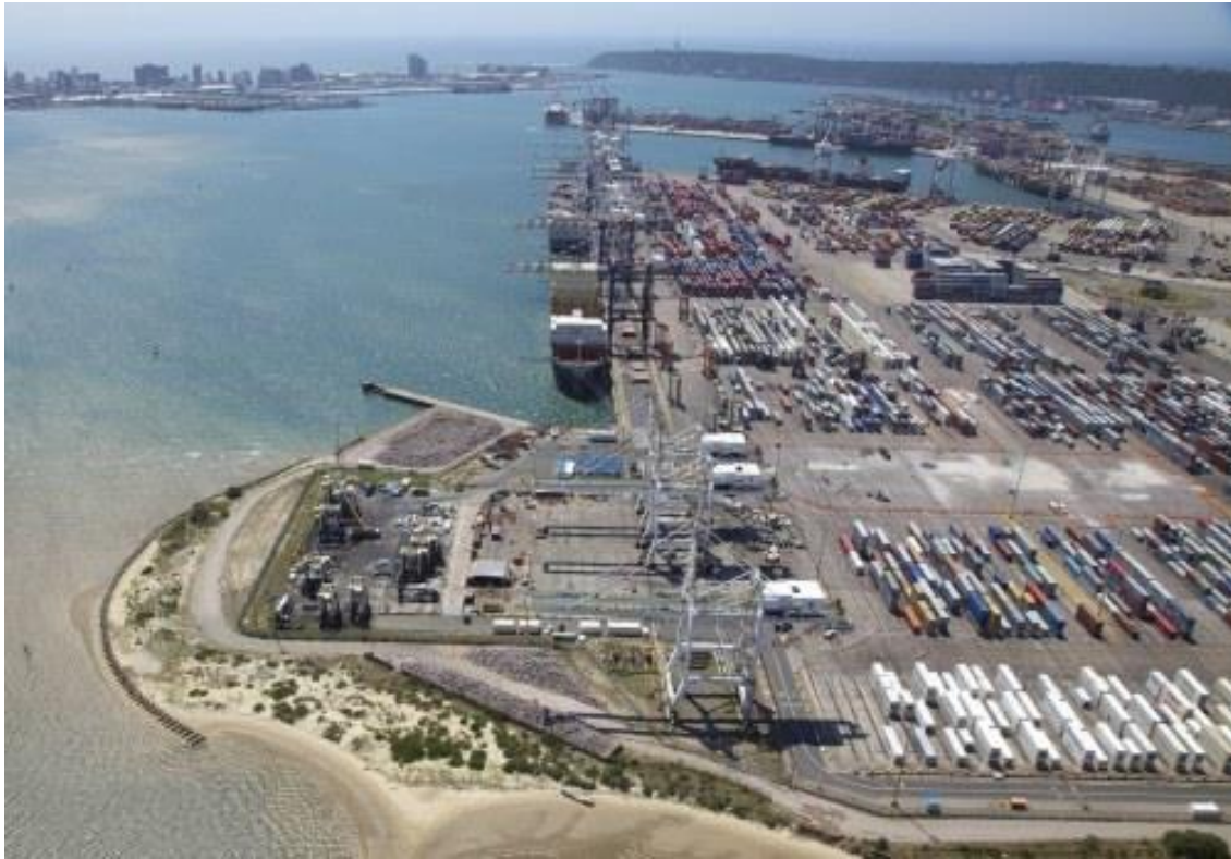
Durban Container Terminal Pier 2 North Quay looking East
